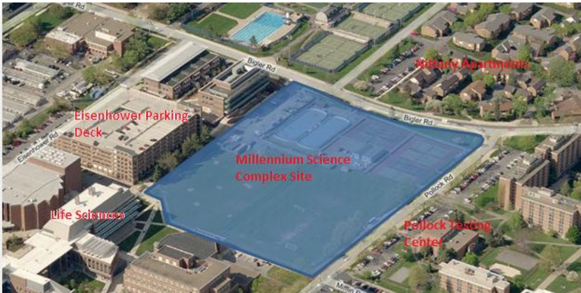
Figure 2.8: Bing Maps View of Millennium Science Complex Site
